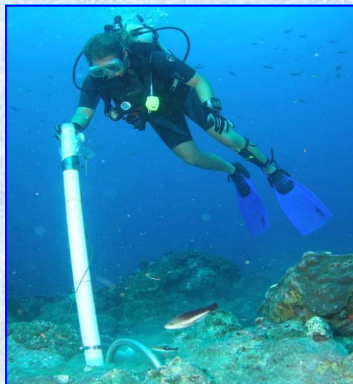
NOAA Working Diver LTJG Tracy Hamburger empties a tube of cement into a newly drilled mooring at the Flower Garden Banks. By Emma Hickerson, UDS
