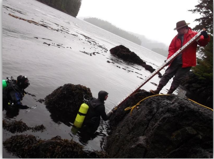
NOAA Divers stationed aboard the NOAA Ship Rainier work to install a tide gauge. (Photo Credit – Mike Gonsalves)
