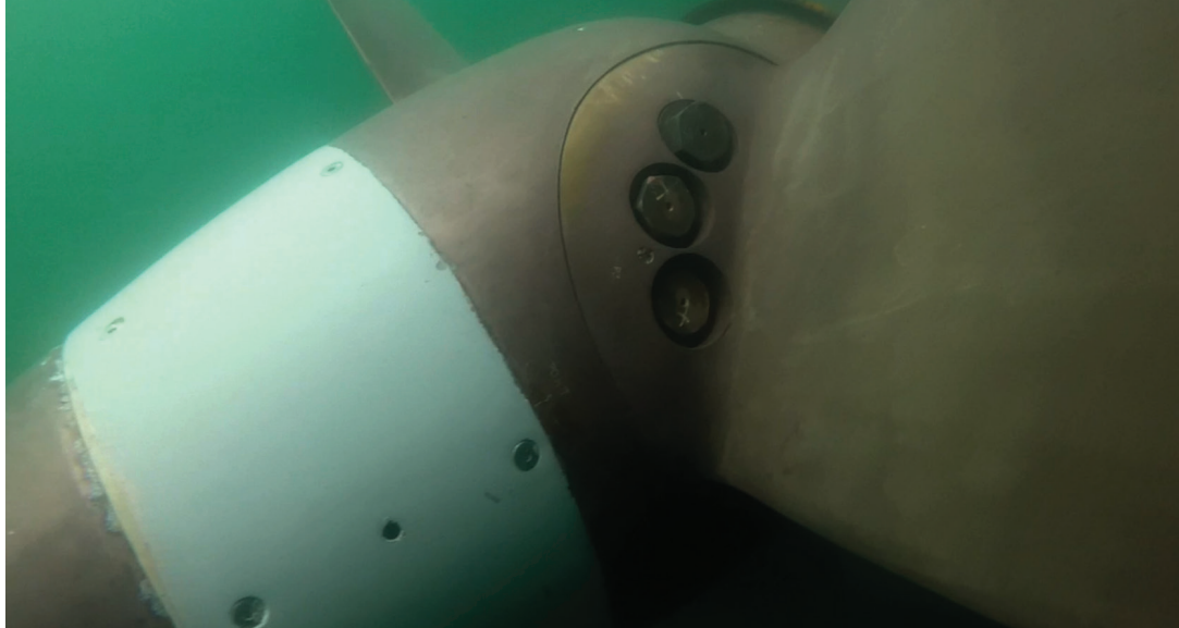
One of the propellers from the NOAA Ship Fairweather , documented during a hull inspection by unit divers. LT Ryan Wartick/NOAA
