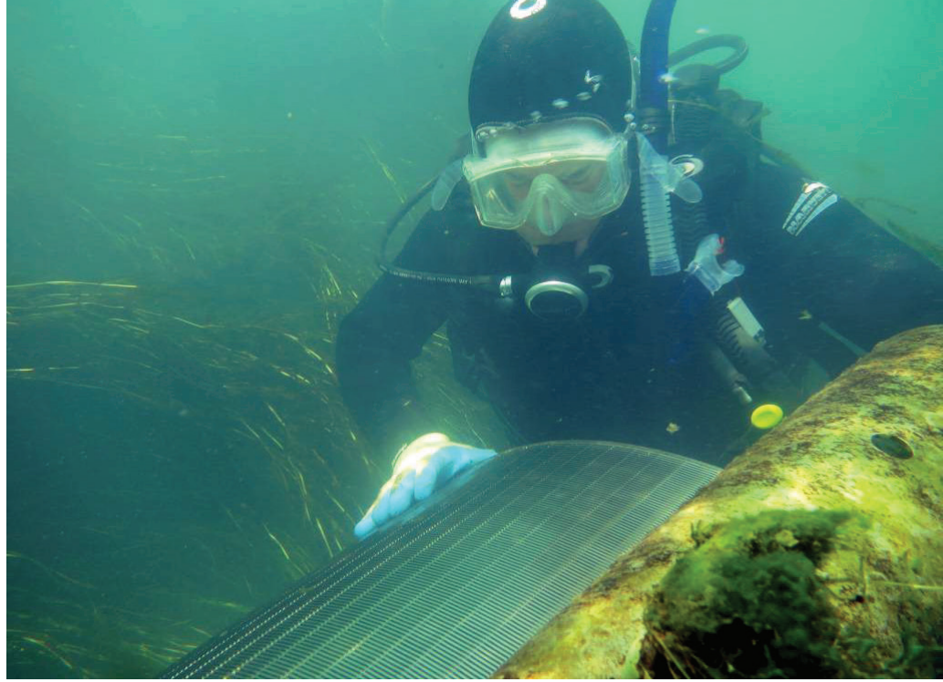
NOAA Diver David White, an engineer at the Santa Rosa unit, inspects a fish screen on a municipal water intake for the City of Redding on the Sacramento River. Steve Thomas/NOAA
