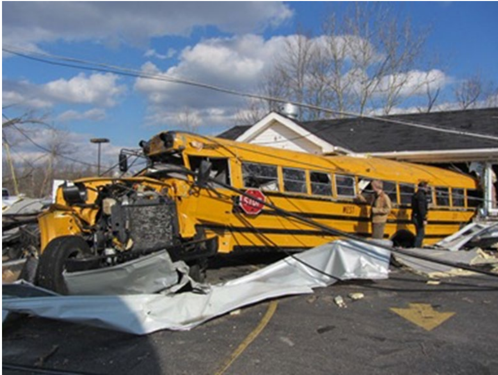
Figure 1: Tornado damage March 2, 2012, in Henryville, Indiana. Damage assessment and area access will benefit from the use of drones once implemented (Credit: NWS Louisville Storm Survey Team).
