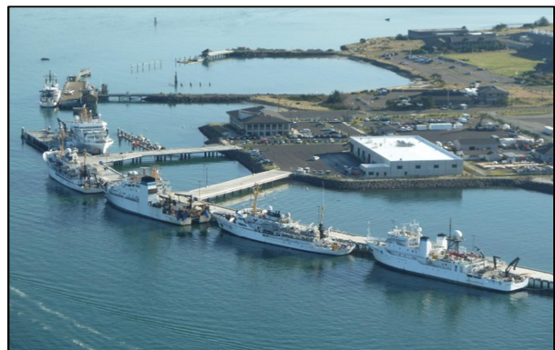
Science, operations, and partnerships come together at OMAO. The NOAA Marine Operations Center-Pacific and Oregon State University's Hatfield Marine Science Center in Newport, Oregon, are pictured here.
