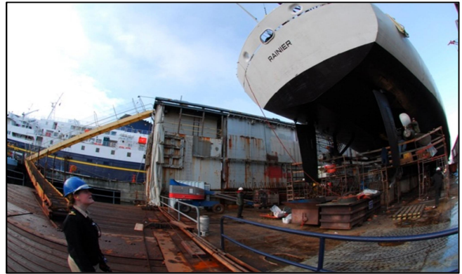
OMAO will adopt a new strategy for managing the lifecycle of ships, aircraft and other platforms. Pictured here is NOAA Ship Rainier undergoing repairs in dry dock.
