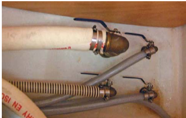
Sea cocks with double clamps – It's important to check for free movement and handle orientation to ensure full travel from opened to closed. Regarding double clamps, remember that the ABYC does not require this in H-27. In fact, if the barb on the thru-hull is not long enough to accommodate the full bandwidth of the clamps, double clamping can cause more harm than good.
